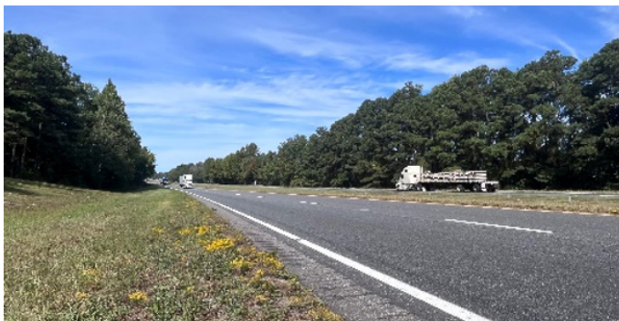
Microsurfacing on US 74 in Scotland County; paved in Fall of 2021
